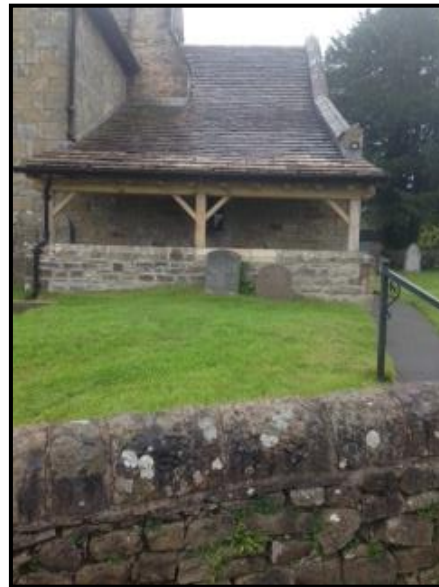
The new roof over the cellar steps
